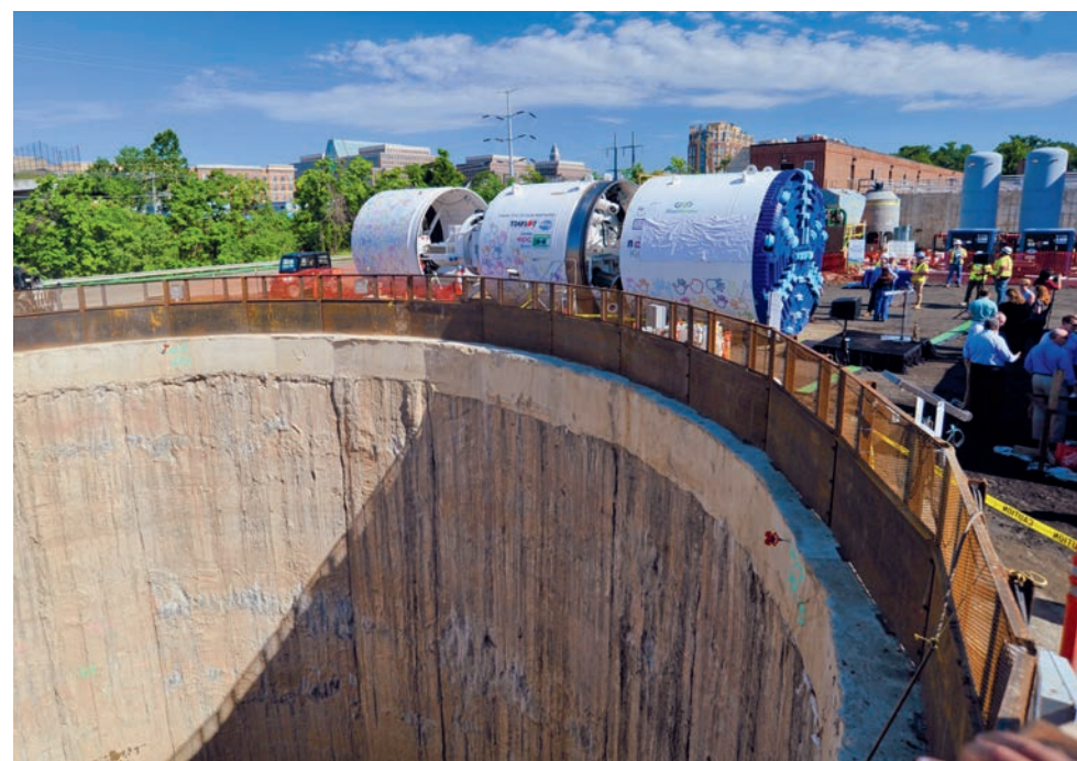
A new tunnel-boring machine sits beside one of two wide shafts that will help reduce sewage-stormwater overflows in Alexandria, VA. One shaft will be used to lower the tunnel-boring machine into place, and the other will carry excavated earth back to the surface. (Whitney Pipkin)
