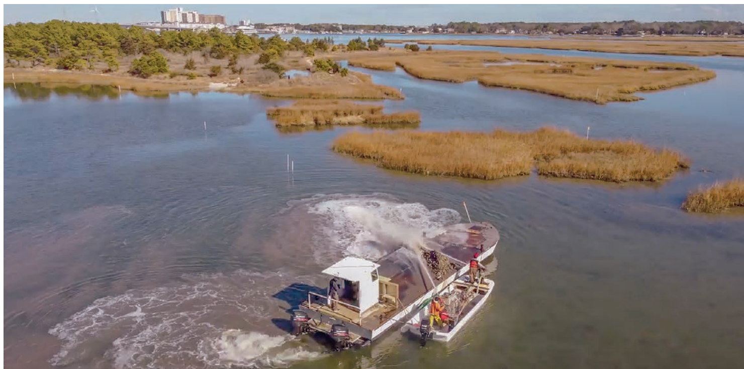
Recycled concrete is sprayed into a tributary of Virginia's Lynnhaven River to form the base of new oyster reefs in February 2022. (Courtesy of Lynnhaven River Now)
