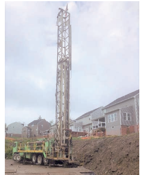
Workers plug an abandoned gas well that was leaking explosive methane into a stormwater impoundment surrounded by homes. (Pennsylvania Department of Environmental Protection)
