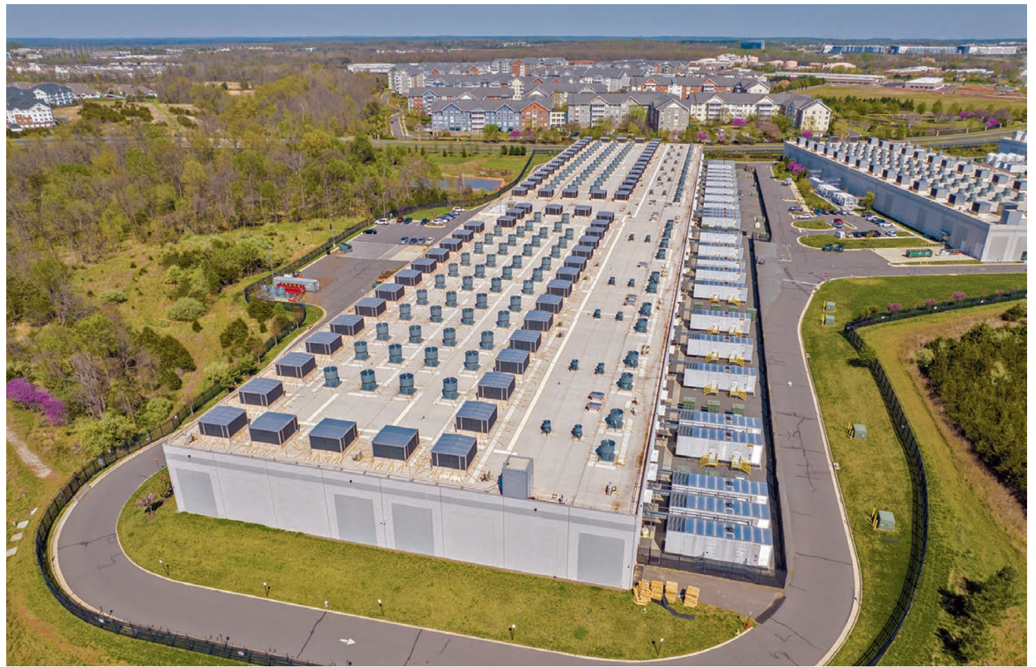
The tractor-trailer-size boxes alongside the this data center in Loudoun County, VA, are backup power generators. (Hugh Kenny/Piedmont Environmental Center)
