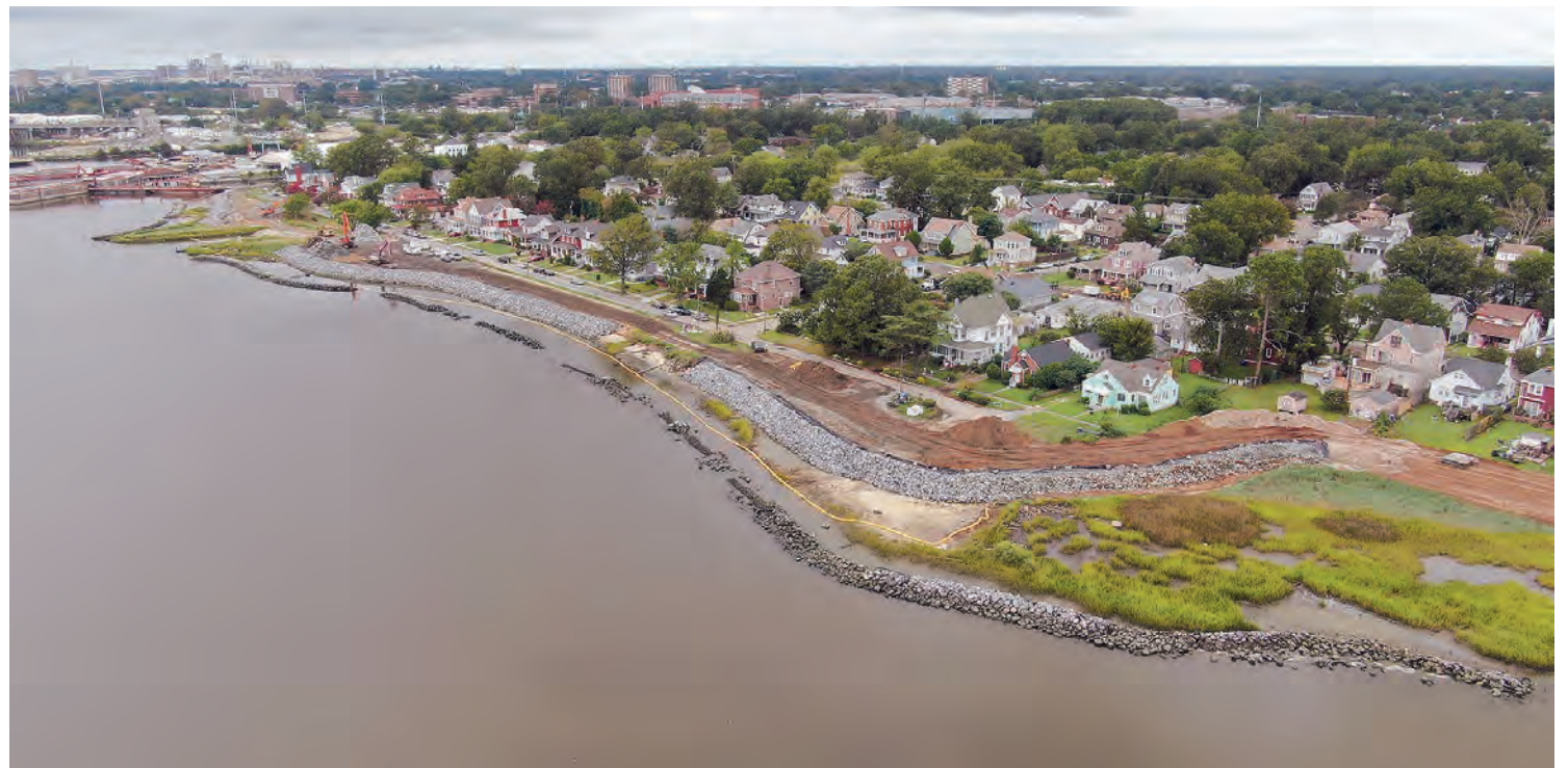
The floodwall built in Norfolk to shield the Chesterfield Heights and Grandy Village neighborhoods from tidal flooding is shown here under construction in October 2020. (Courtesy of the city of Norfolk)
