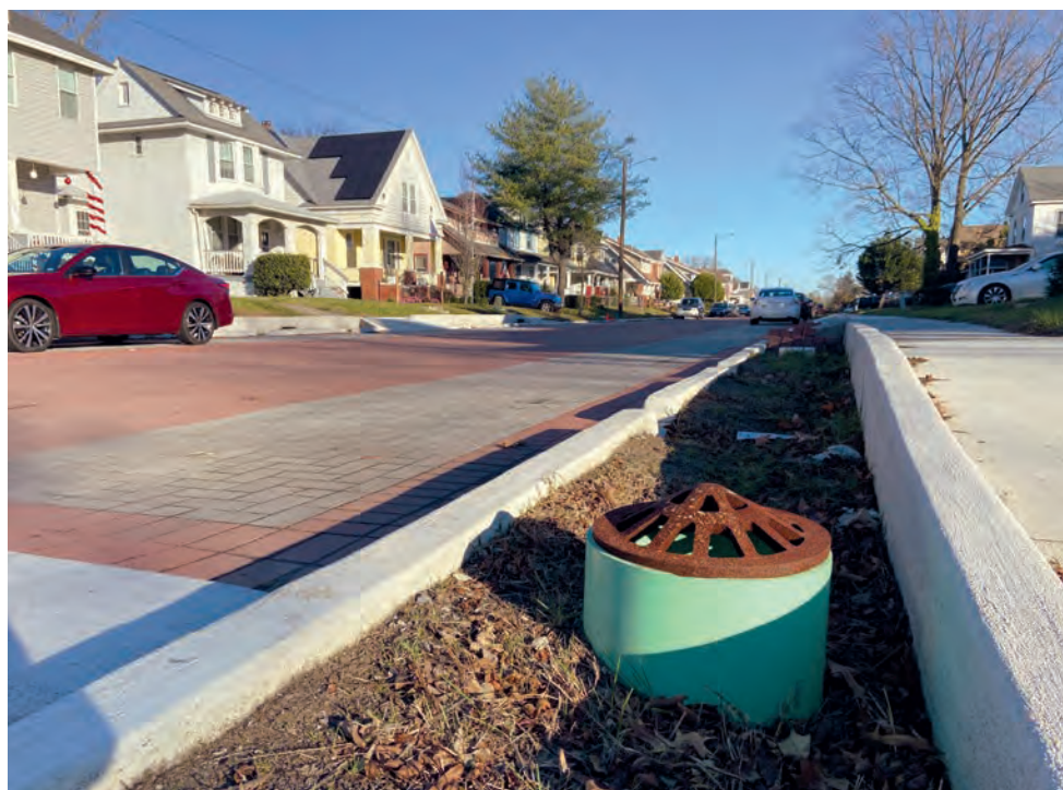
In Norfolk's Chesterfield Heights neighborhood, a newly installed bioswale is designed to capture and treat stormwater before it reaches the Eastern Branch of the Elizabeth River. Meanwhile, new permeable pavers allow water to soak into the ground beneath the street. (Jeremy Cox)
