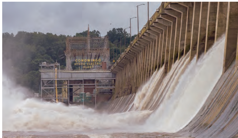
Conowingo was built in 1928 to generate electricity, and it inadvertently acted as a trap for nutrient and sediment pollution flowing downstream to the Chesapeake Bay. Over the years, sediment buildup behind the dam has reduced its pollution-trapping capacity. (Dave Harp)
