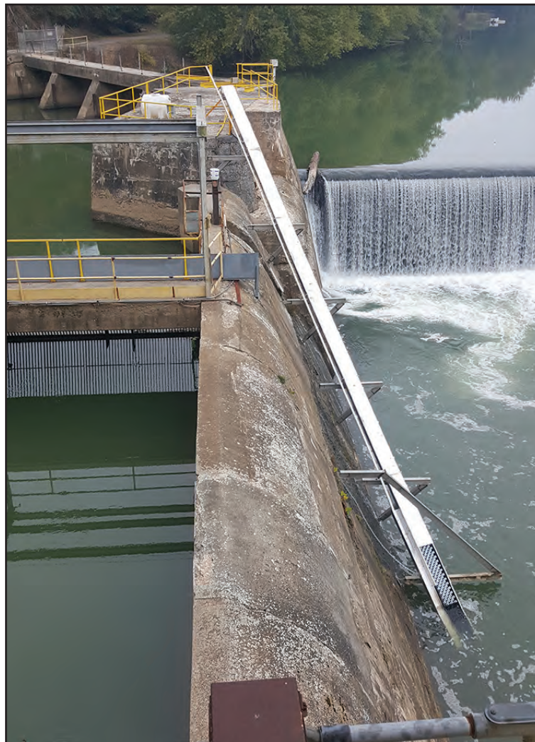
This eelway, installed in 2019, will help immature American eels get past Dam #5 near Falling Waters, WV, on the Potomac River. (David Sutherland / U.S. Fish and Wildlife Service)
