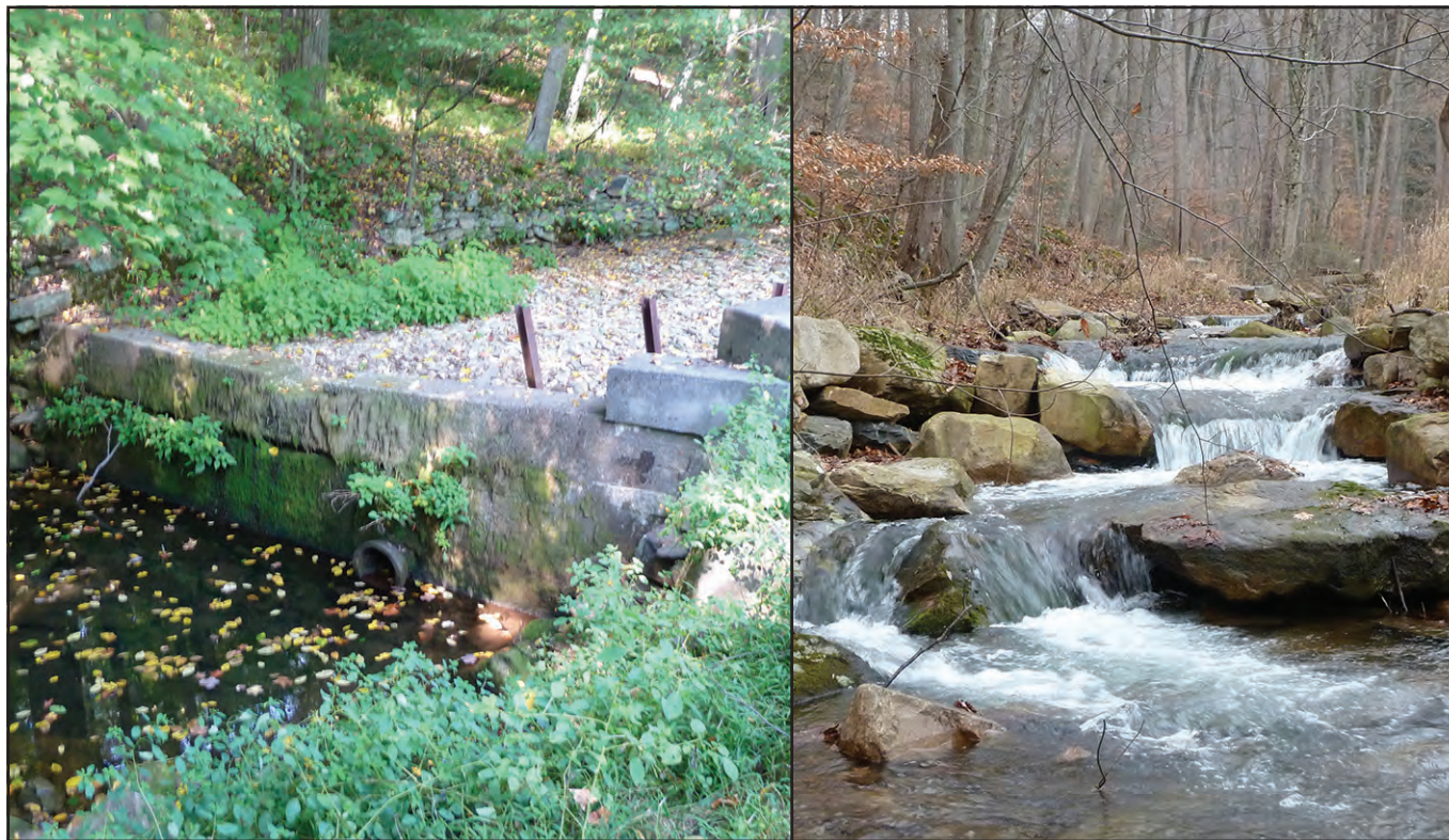
These photos show Clifford Branch in Frederick County, MD, before and after a culvert was removed in 2017. A dam, 2 miles downstream, was removed in 2012. The two projects will allow brook trout and other native fish passage on the waterway. (Mark Secrist / U.S. Fish and Wildlife Service)
