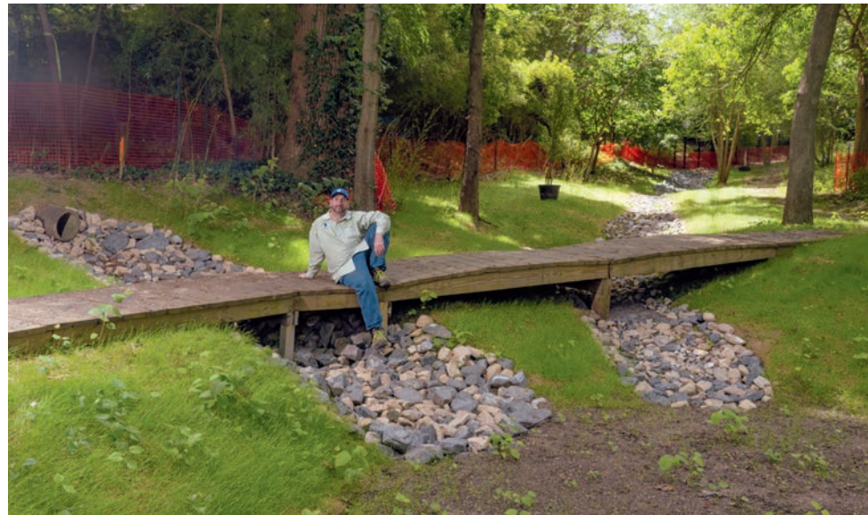
Ben Fertig of the Severn River Association sits near “step pools” in Annapolis’s Wardour neighborhood, which are designed to slow down and absorb stormwater. (Dave Harp)
