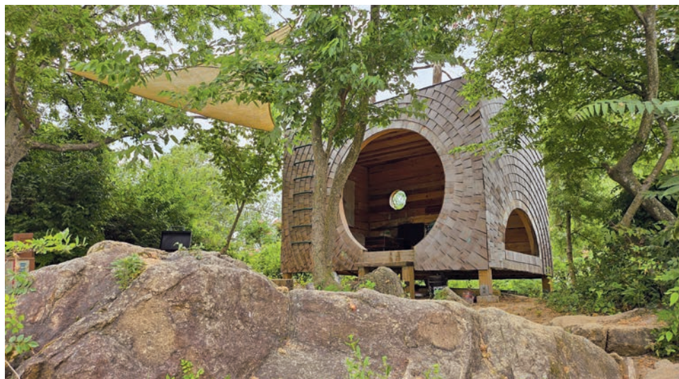
This shelter, available to rent on Sharp's Island in Richmond, is the third built there by current owners. Flooding washed away the previous two attempts. (Lauren Hines-Acosta)
