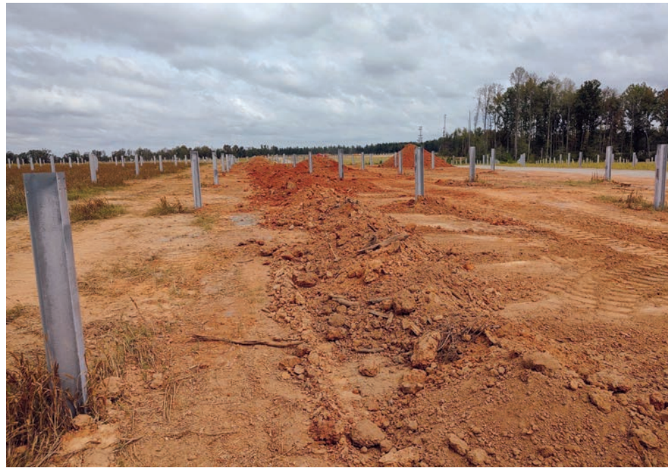
Moving and grading soil during the construction of solar energy sites can lead to erosion and increased stormwater runoff. (landrehab.org/solar-farms)
