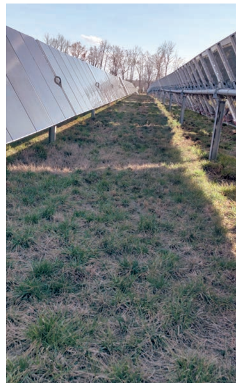
Post-construction efforts to seed the land at this Virginia solar farm, shown here in midwinter, enjoyed relative success. The work also met the state's minimum standards for erosion and sediment control. (landrehab.org/solar-farms)
