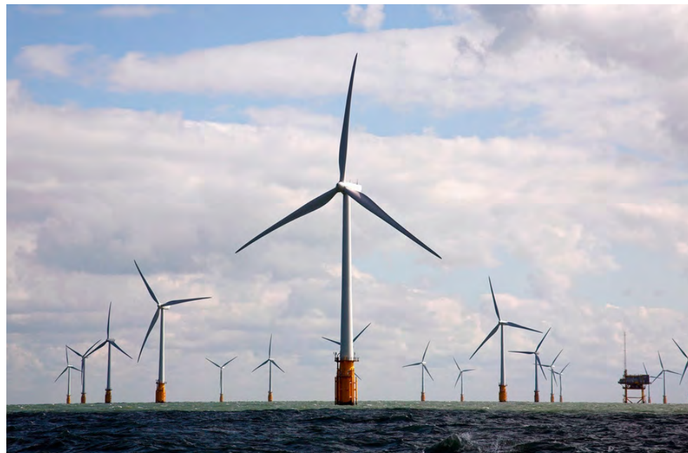
Proposals for wind energy projects offshore of Ocean City, MD, have drawn both opposition and support. The Thanet Wind Farm, shown here, consists of 100 turbines located about 7 miles offshore of England. (Vattenfall Nederland)
