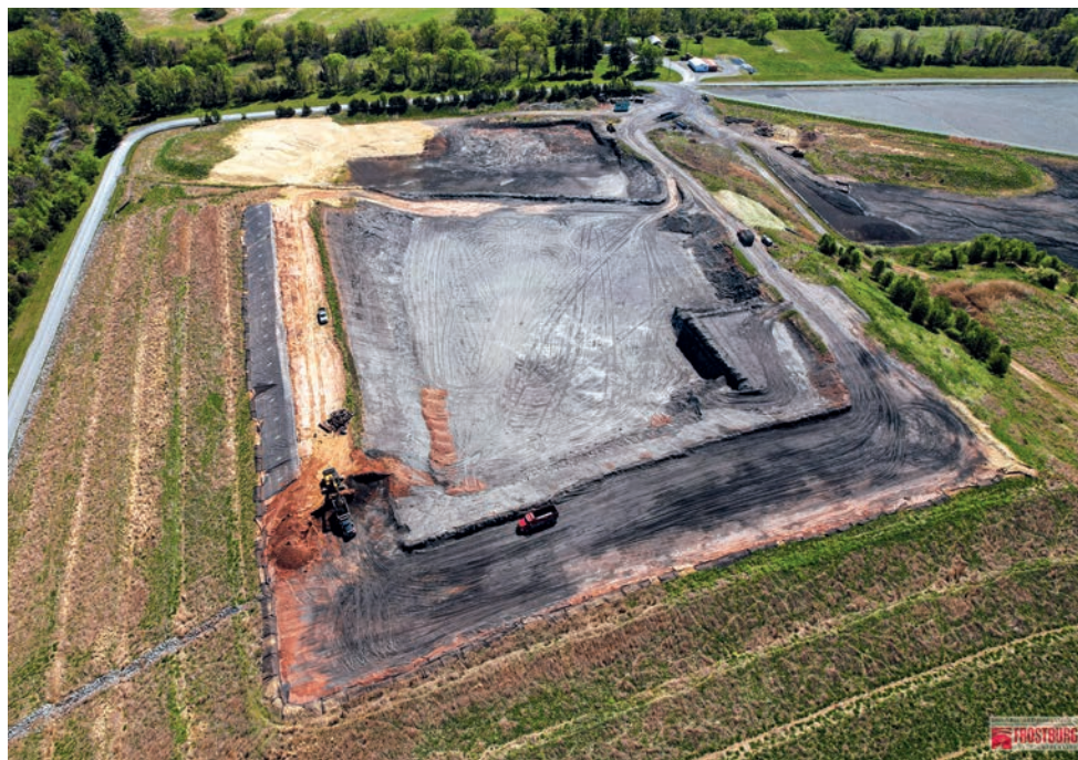
More than 850,000 tons of coal ash have been excavated from the Westland coal ash landfill near the Potomac River in Montgomery County, MD, and used to make cement. (Courtesy of Frostburg State University)
