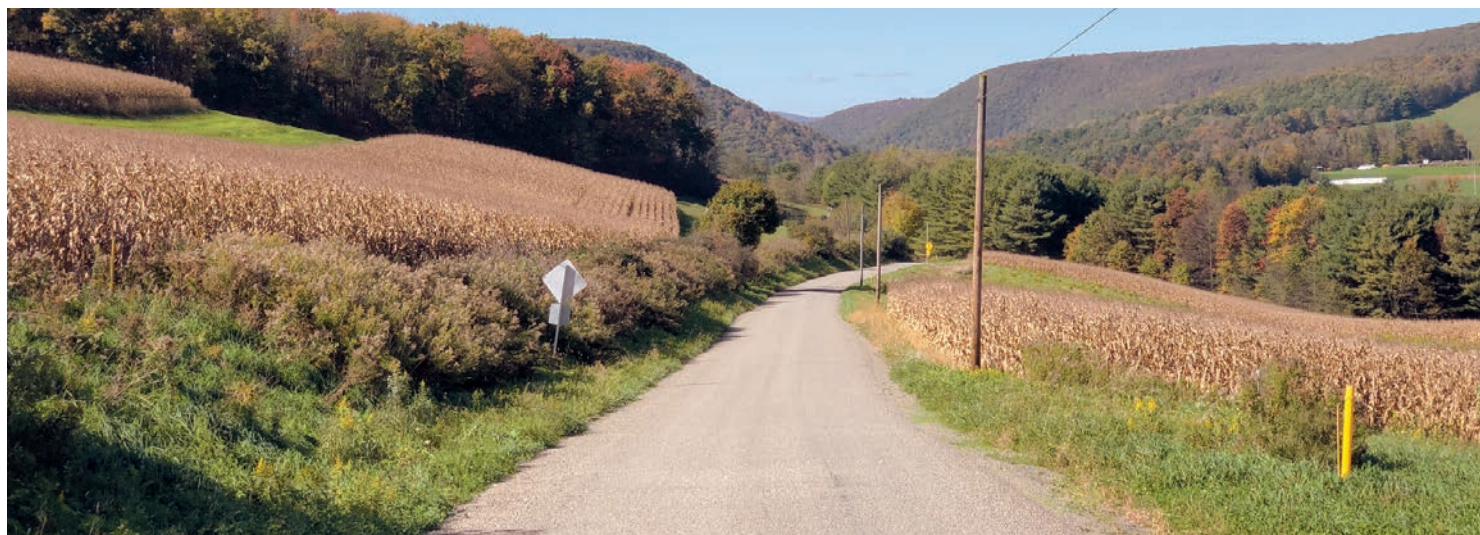
Lick Run Road in Lycoming County, PA, north of Williamsport, makes up part of the roughly 25,000 miles of dirt or gravel roads in the state. (famartin/CC BY-SA 4.0)
