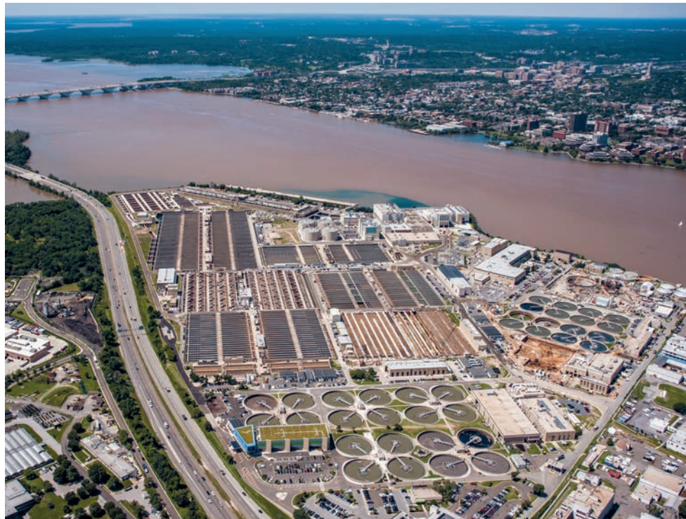
The Blue Plains Advanced Wastewater Treatment Plant is very effective at removing nutrient pollution from wastewater, but it's an energy-intensive process. (Courtesy of DC Water)
