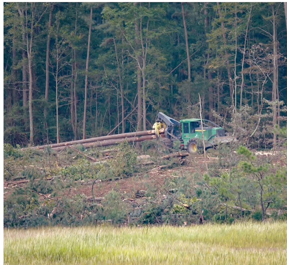
Equipment is seen among a portion of the land at Virginia's Camp Peary where trees were removed. No vegetated riparian buffer was retained between the cleared area and the adjoining marsh. (Dave Malmquist)
