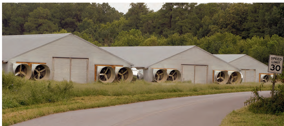
A trio of chicken houses near a road on Maryland's lower Eastern Shore feature giant exhaust fans that pump ammonia-laden air out of the buildings. (Dave Harp)
