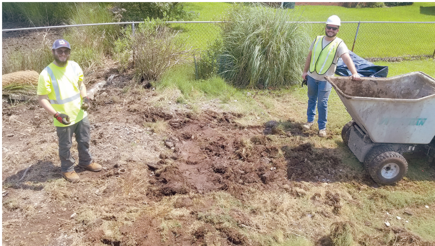
Frederick Schroeder of the Elizabeth River Project, left, works with the James River Association's Ryan Walsh to bring clean sand to an excavated rubble area along the Lafayette River, creating a new living shoreline. (Elizabeth River Project)
