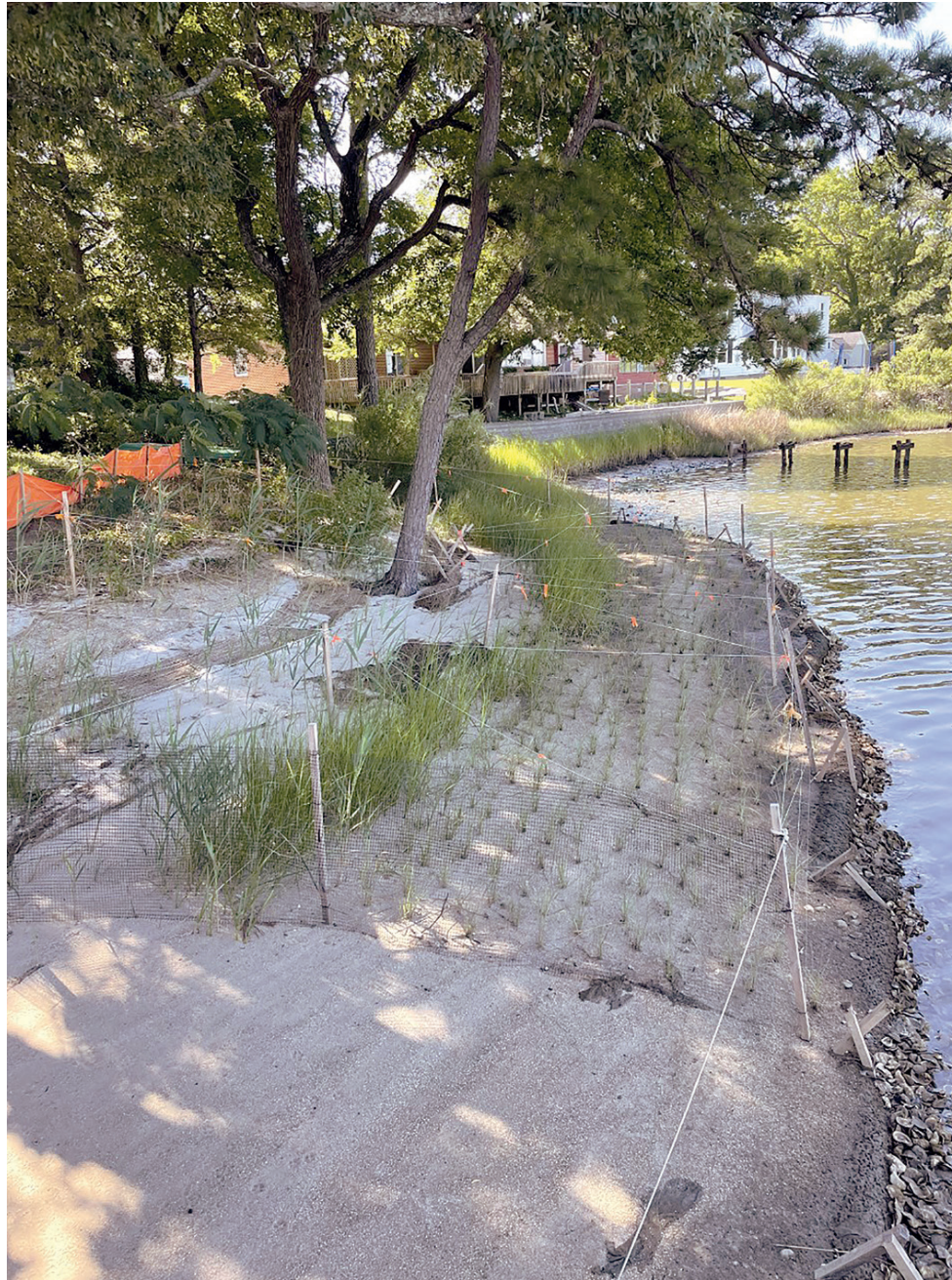
Living shorelines, like this newly created one on a Virginia property, use nature-based solutions to help control erosion and provide wildlife habitat. (Sterling Rollings)
