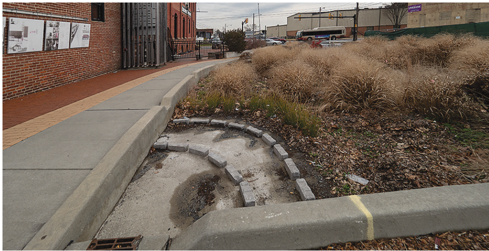
A rain garden installed along the Lancaster Brewing Company in Lancaster, PA, is designed to reduce the amount of water traveling through underground pipes by capturing and absorbing some of the stormwater runoff before it enters the system. (Dave Harp)
