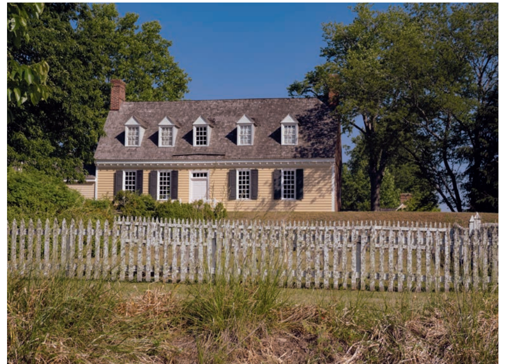
The Long Hill plantation house, built in the mid-1700s, will be part of the new Wetipquin Creek State Park on Maryland's Eastern Shore. (Dave Harp)
