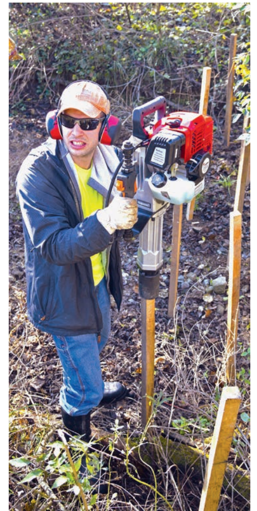
Matt Wilson of Susquehanna University's Freshwater Research Institute uses a power tool to pound posts into a streambed to help create an artificial beaver dam. (Ad Crable)
