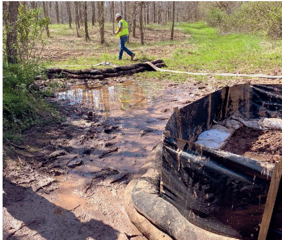
Sediment-laden water escapes a containment area in April after a "frac-out" at the QLoop fiber-optic line construction site in Frederick County, MD. (Maryland Department of the Environment)
