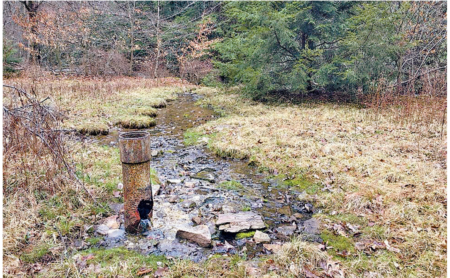
This abandoned gas well in Pennsylvania was eventually plugged after a petroleum sheen was found flowing into a tributary of the West Branch of the Susquehanna River. (Pennsylvania Department of Environmental Protection)
