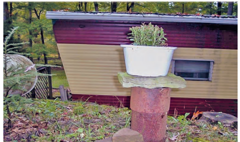
A stone and flower pot were placed on this abandoned oil and gas well to stop emissions, ineffectively, near a mobile home. (Pennsylvania Department of Environmental Protection)
