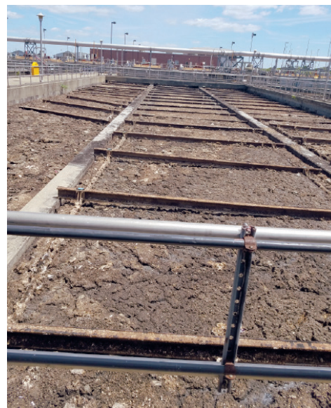
This photo from the state inspection report for the Patapsco Wastewater Treatment Plant in Baltimore shows settling tanks rendered inoperable by an accumulation of solids, fats, oils and grease. (Maryland Department of the Environment)
