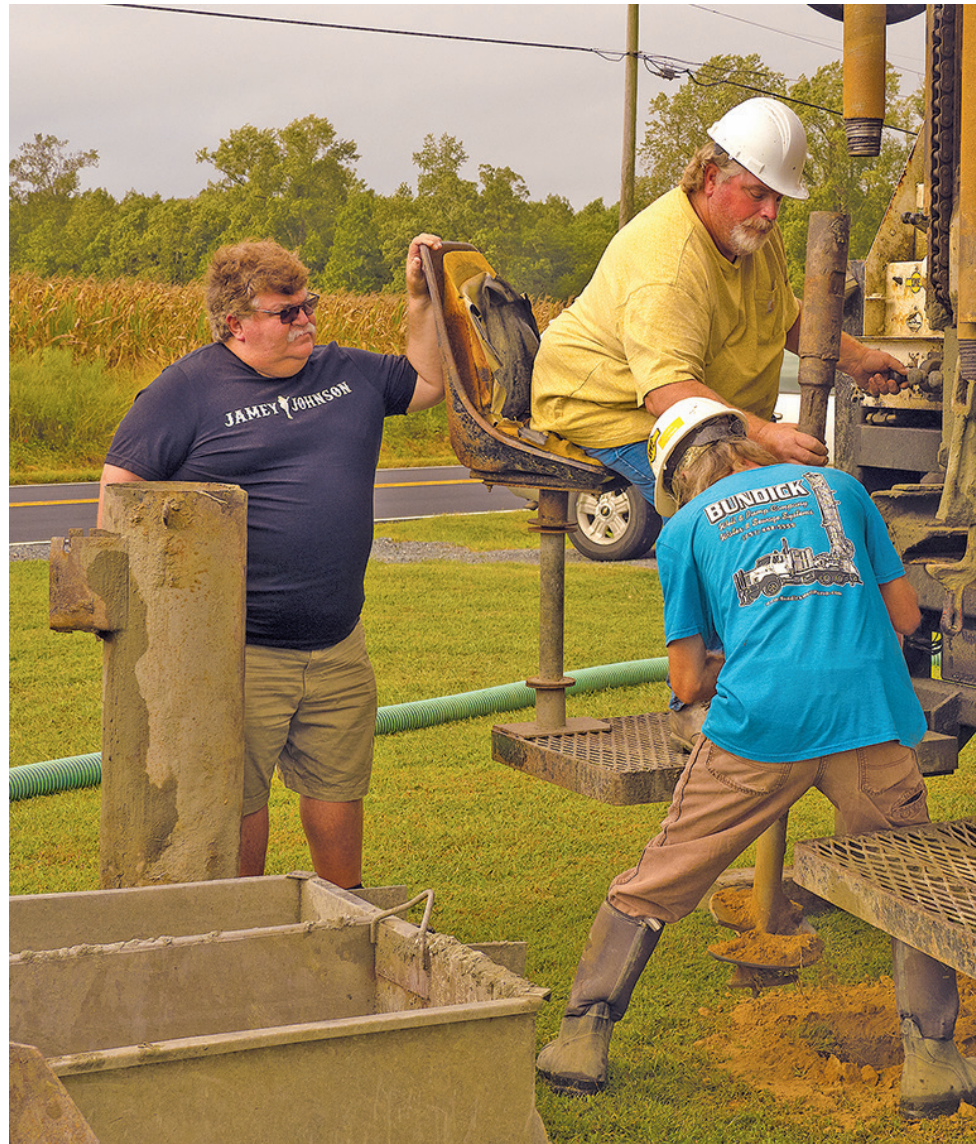
Danny Bundick of the Bundick Well & Pump Company looks on as driller Jerry Fisher, center, and assistant Ben Privegen drill a well into the Yorktown-Eastover aquifer near Chincoteague, VA. (Dave Harp)
