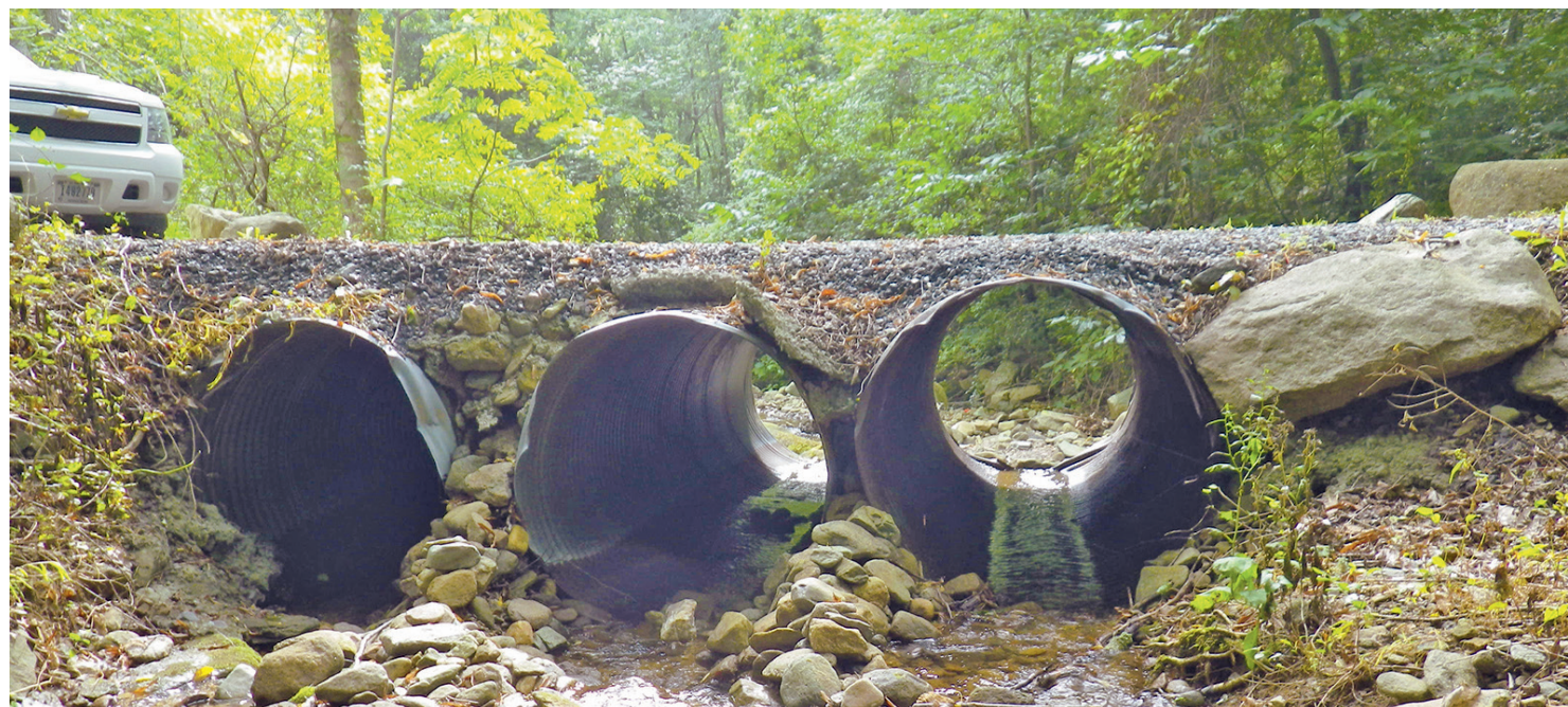
Culverts should be designed not only to avoid flooding but also to allow the passage of aquatic life. This less-than-ideally designed culvert on a Rappahannock River tributary was replaced with a steel bridge that allowed the stream to pass naturally underneath it. (Ben Hutzel, U.S. Fish and Wildlife Service)
