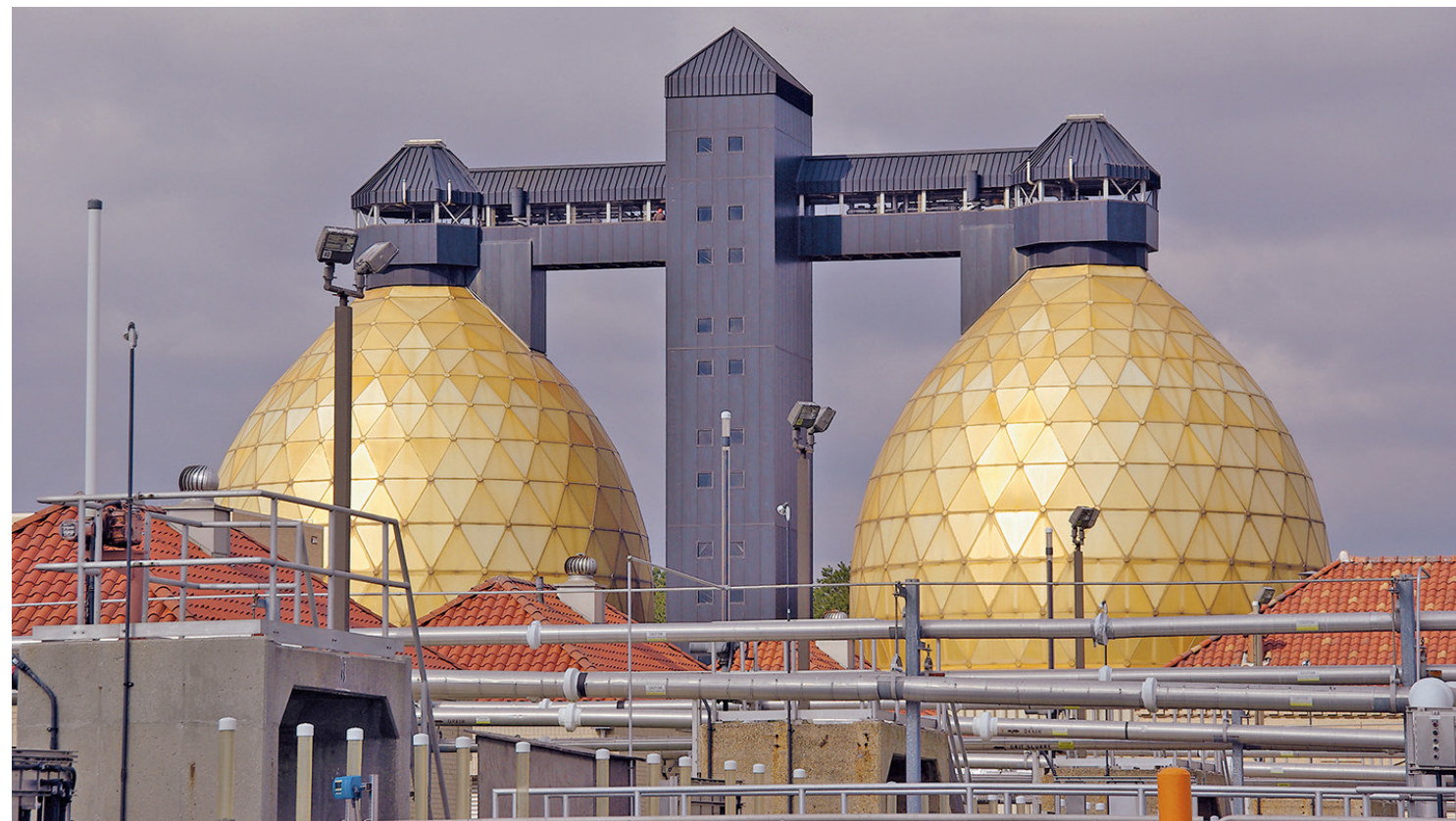
The Back River Wastewater Treatment Plant in Baltimore County, MD, features a distinctive gold-domed pair of anaerobic digesters used to process sewage sludge. (Kristian Bjornard/Wikimedia Commons)
