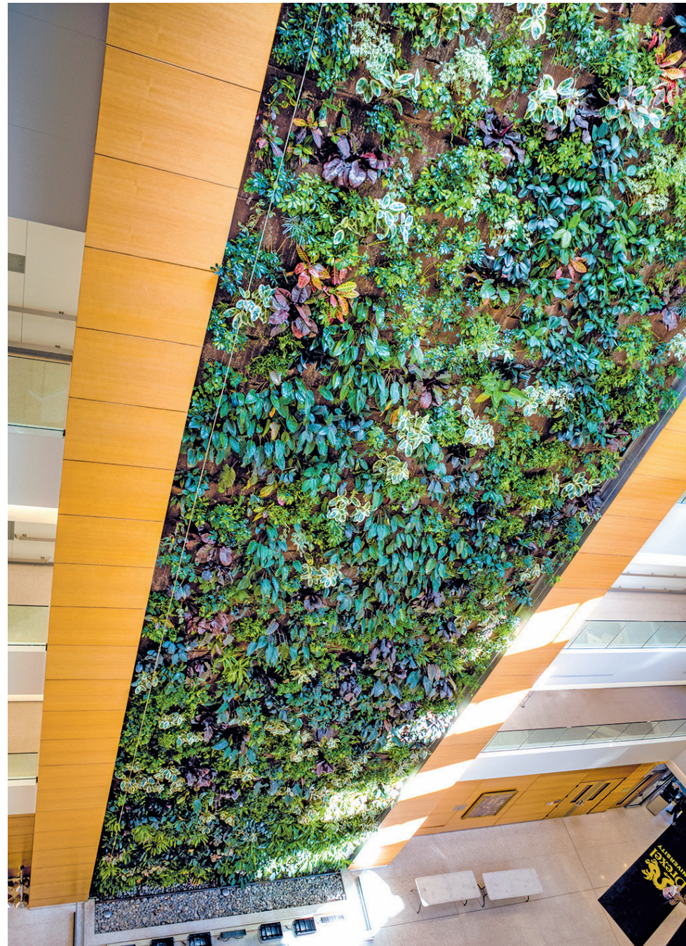
The Papadakis Integrated Science Building at Drexel University in Philadelphia features a “living wall.” (Terry Robinson, CC BY-SA 2.0)
