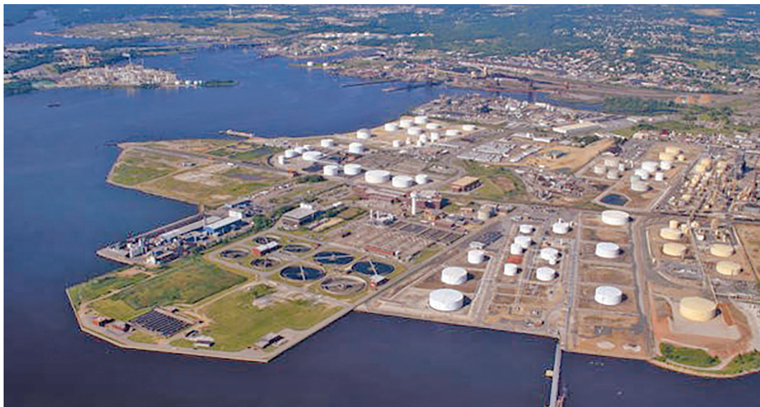
Baltimore's Patapsco Wastewater Treatment Plant, in left foreground, discharges about 55 million gallons of treated wastewater daily into the Patapsco River just upriver of the Key Bridge. (Jane Thomas/Integration and Application Network, UMCES)
