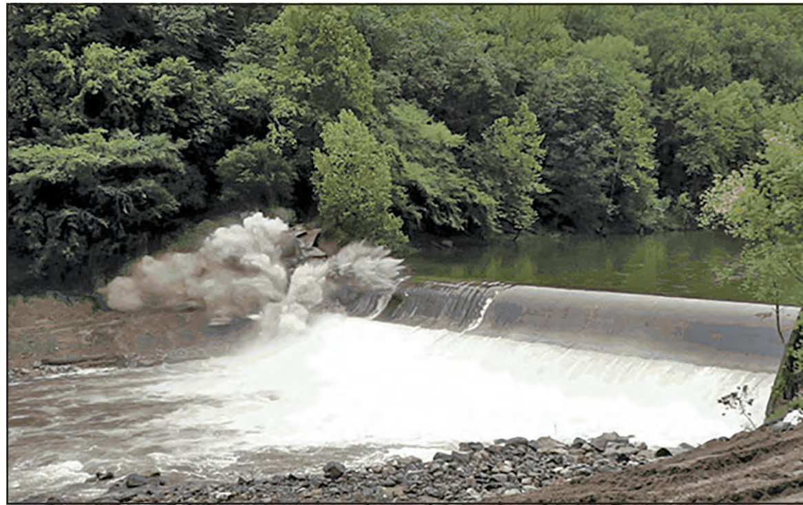
Explosives breach the Bloede Dam on Maryland's Patapsco River in September, the beginning of a demolition process that will open upstream habitat to migrating fish and eels. (MD DNR)
