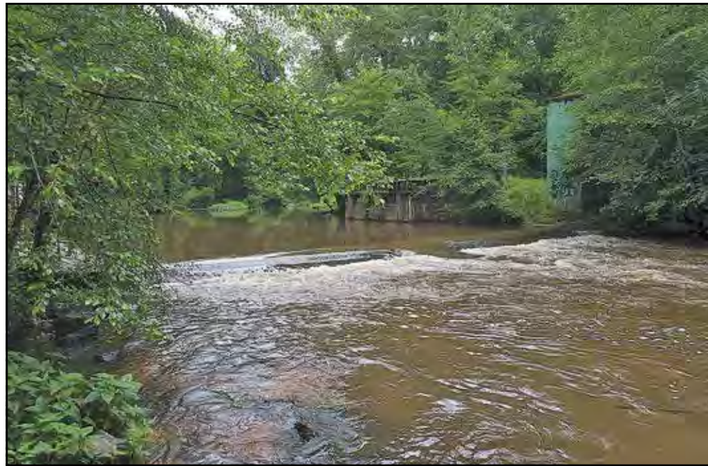
Water flows over the weir at the USGS gaging station on the upper Choptank River at Red Bridges. This photo was taken at 10 a.m. on June 19, when the flow was approximately 130 cubic feet per second after two days of thunderstorms. (Dave Harp)
