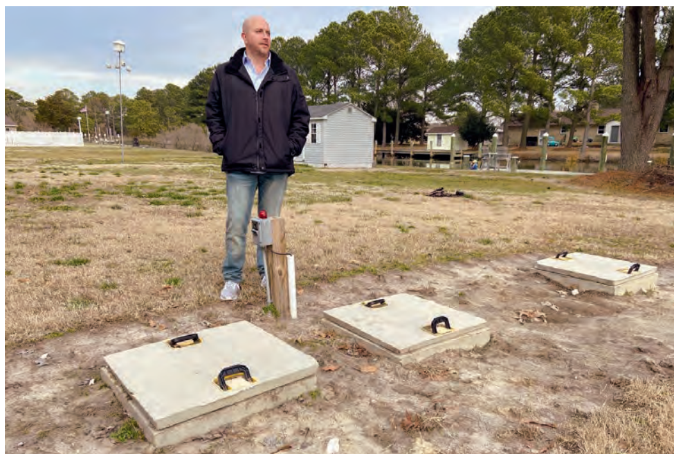
Andrew Karolick stands beside lids to the holding tanks at his house near Crisfield, MD. He and his family use paper plates and avoid doing laundry to keep the tanks from filling too quickly. (Jeremy Cox)
