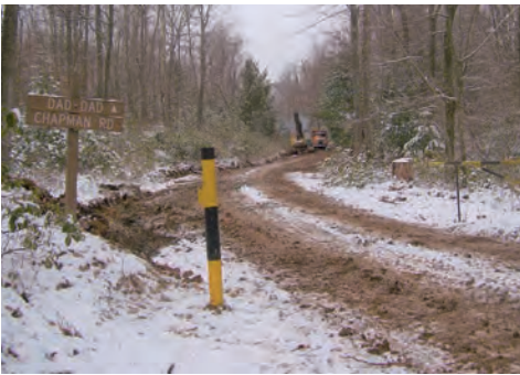
A dirt road and trail in the Loyalsock State Forest in Pennsylvania is converted into an access road for two well pads that support fracking for natural gas. (Barbara Jarmoska)
