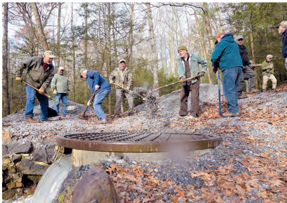
Volunteers with the Doc Fritchey Chapter of Trout Unlimited heave limestone into a doser so that trout can live in about 20 miles of Stony Creek, Pennsylvania's first designated scenic river. (Ad Crable)
