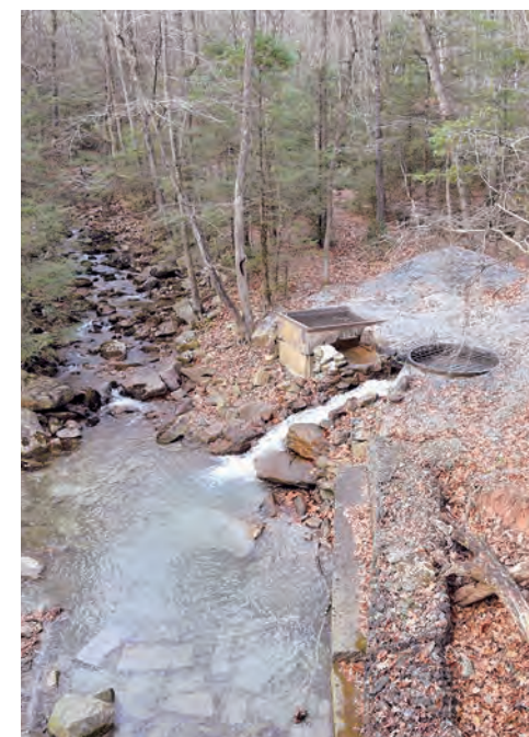
This manually operated limestone doser on Rausch Creek in Pennsylvania neutralizes acidity that lingers from past coal mining and would otherwise devastate fish habitat. (Ad Crable)
