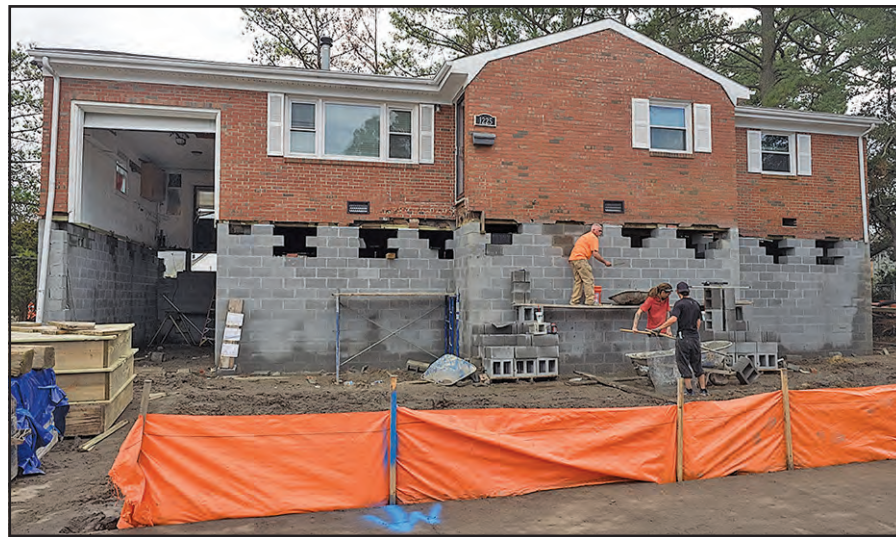
Masons fill in holes from steel beams used to raise a house in the Larchmont neighborhood of Norfolk, VA. The Lafayette River often floods the area. (Dave Harp)
