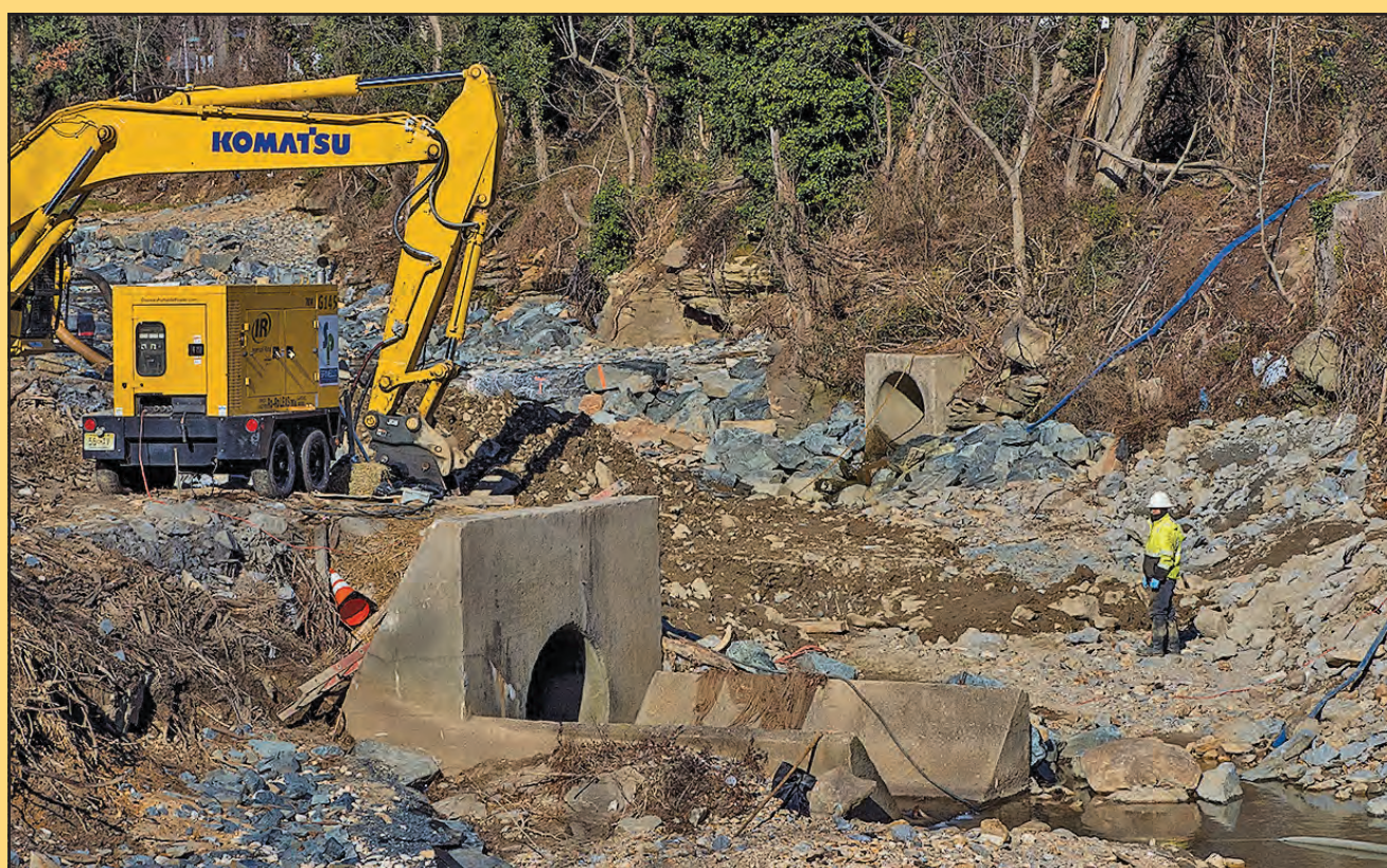
Construction crews restore Chinguapin Run in Baltimore city, moving sewer line out of a channel and stabilizing banks. Trees planted along stream by volunteers were taken out, but officials say the reductions in erosion and sewage leaks outweigh the loss. (Dave Harp)
