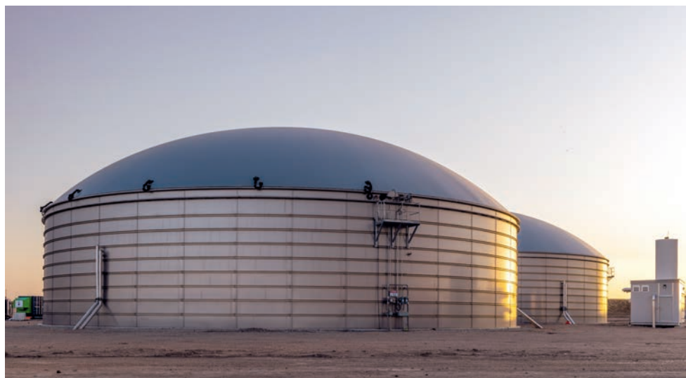
Anaerobic digesters like this one are airtight vessels that capture the methane produced as the bacteria in manure digests organic waste. (Vanguard Renewables)
