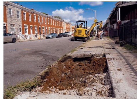
An excavator operated by a crew from Blue Water Baltimore cuts tree pits in 2022 in the concrete sidewalk in Easterwood, a West Baltimore neighborhood near Coppin State University. (Dave Harp)
