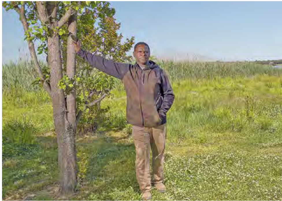
James Jones discovered the culvert dumping stormwater from the Chalk Point power plant into Coleman Creek, lined by the phragmites behind him. His property floods during heavy rains, when Coleman Creek experiences flash floods. (Dave Harp)
