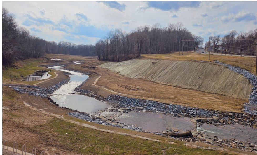
Last year's removal of a dam on Blackwater Creek allowed the city of Lynchburg, VA, to restore the creek's path along what had been the bottom of Lynchburg's College Lake. (Lauren Hines-Acosta)
