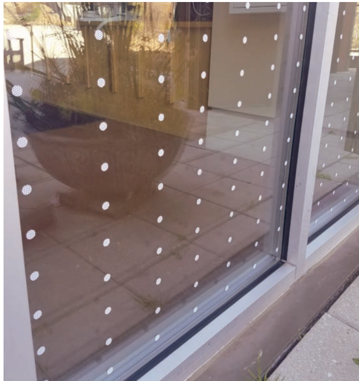
Adhesive stripes or rows of dots on window exteriors drastically reduce bird fatalities from window collisions. (Courtesy of CollidEscape.org)
