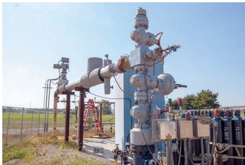
This equipment is part of an underground carbon storage well at an Archer Daniels Midland corn processing and ethanol facility in Decatur, IL. (Courtesy of Archer Daniels Midland)
