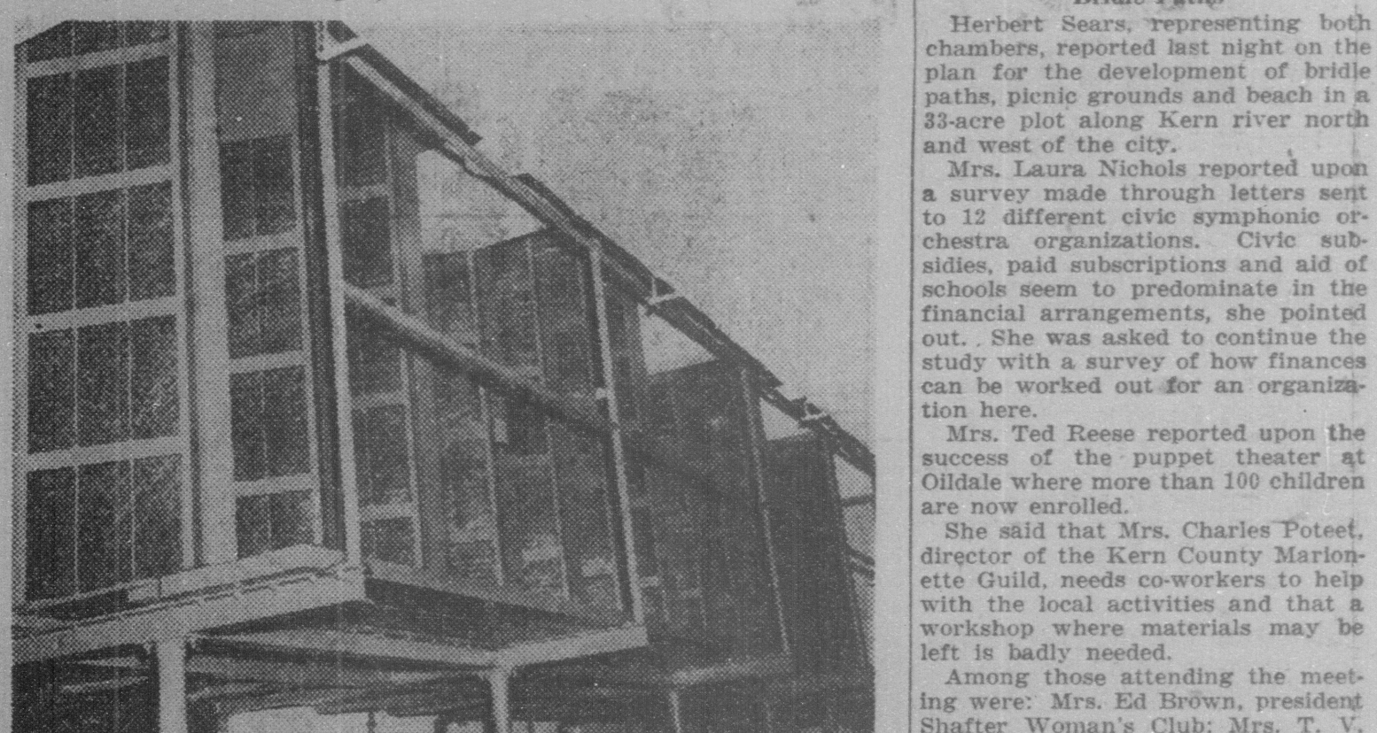
MACHINERY DUSTPROOF—Because huge fans suck out excessive heat generated by the huge voltage used in the 200,000-watt station, these spun glass filters flank the upper part of the pump room, catching all dust particles and preventing them from settling in the delicate equipment of the station. Much dusting is done anyway to keep tubes and coils dust free.
