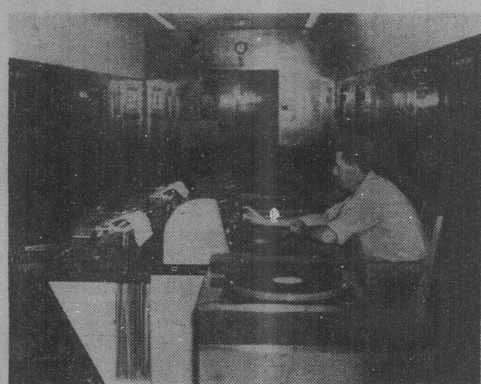
OPERATE CONSOLE—Here is the console table of the big broadcasting station, with W. E. Niehaus, one of the staff engineers, turning the dials that control the audio intake. At this table are kept logs of all incoming programs that are transmitted overseas. Down the length of this 124-foot room are control panels for transmitters and modulators. A "mike" can be fitted into the console table, permitting the operators to talk overseas, but this is never done unless to straighten out mechanical difficulties that arise in transmitting. Engineers have the pride of "the show must go on" in working fast to prevent tangles in the station's operation.
