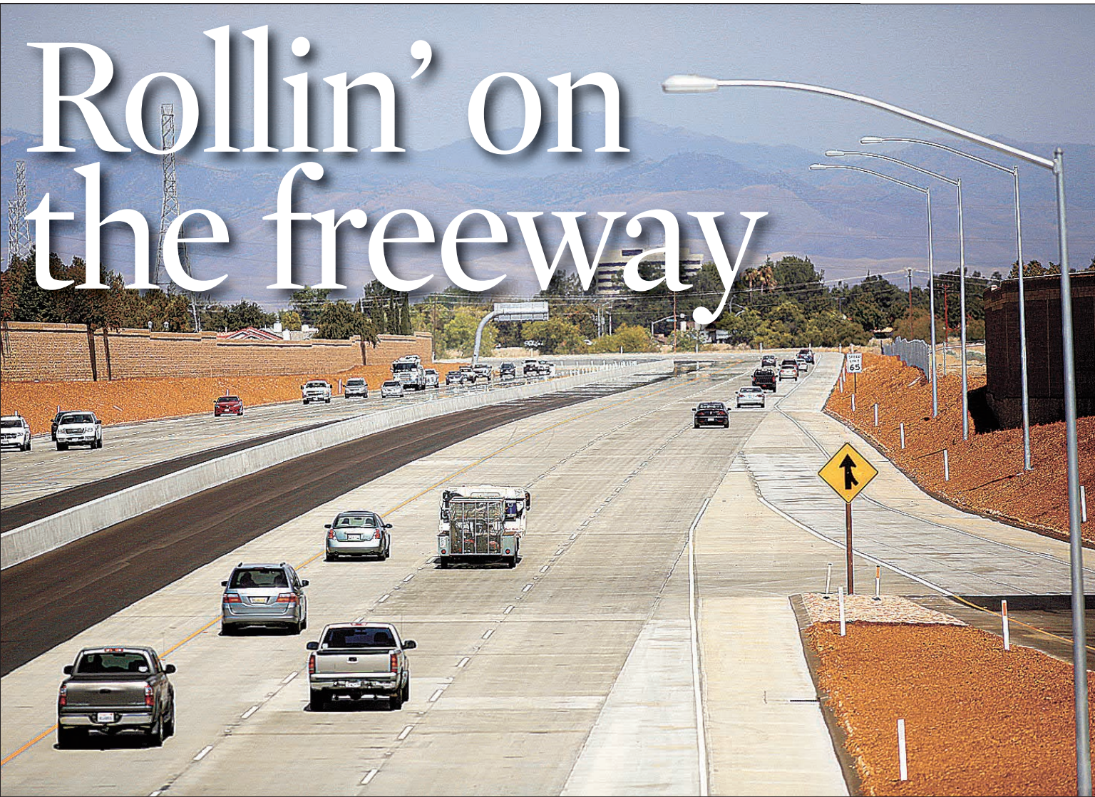
Traffic moves steadily on the new Westside Parkway near Calloway Drive on Friday afternoon. The new east-west freeway, which began to take shape in 2009, extends five miles from Truxtun Avenue to Allen Road.
