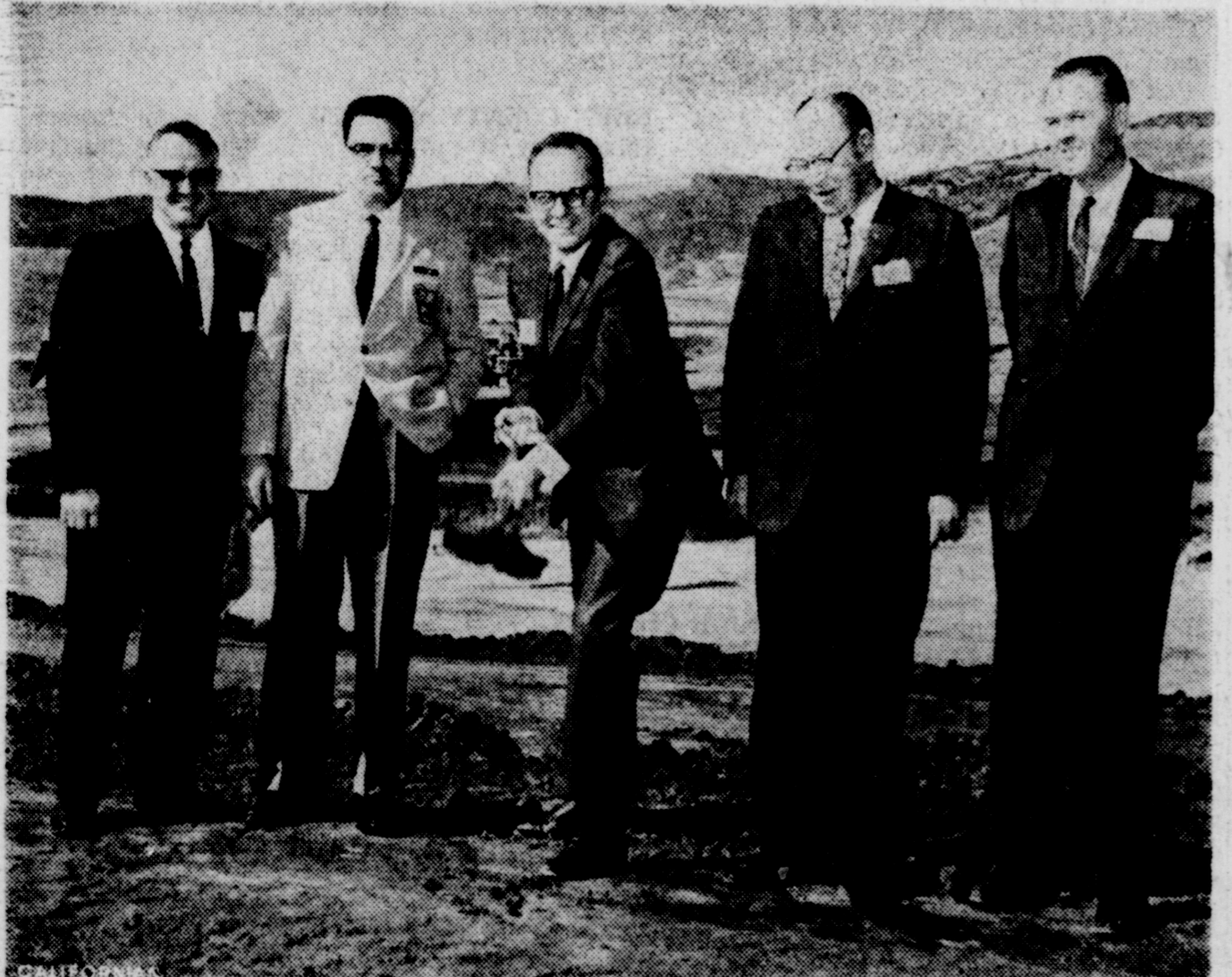
John M. Kinard, president of Pacific Western Industries, heralds start of construction of a $17 million cement plant his firm is building at the southern end of the Tejon Ranch. Flanking him, from the left, are President Alan Pettit of the Kern County Board of Trade; President James Starr of the Antelope Valley Progress Association; Kern County Supervisor John Holt; Duncan Patty, Tejon Ranch vice president in charge of oil and mining. Behind them is the low range of hills which will be the backdrop of the plant, to be completed in about a year.
