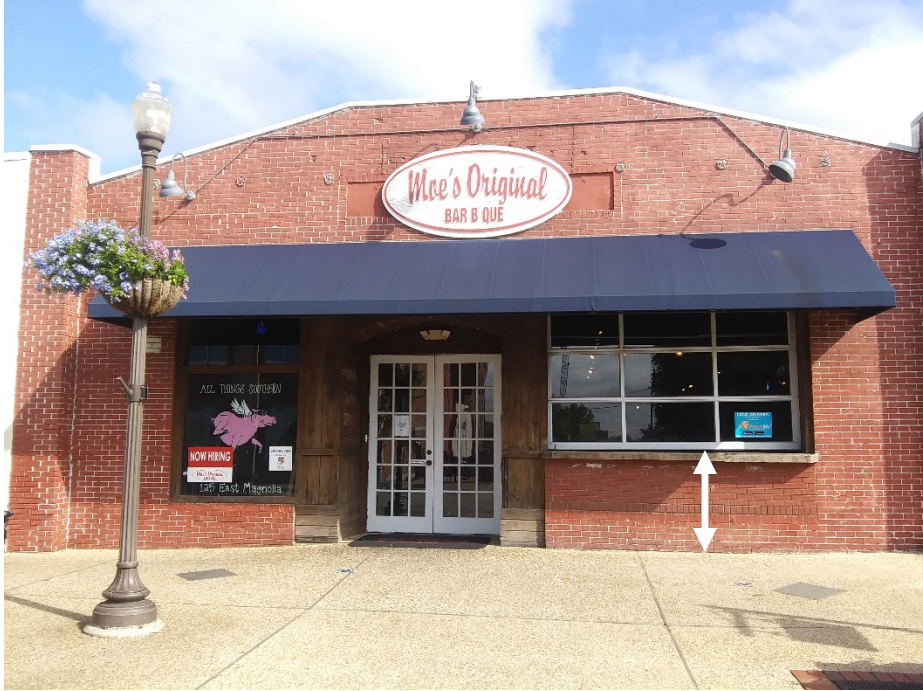
COMPLIANT 3.5' bulkhead
