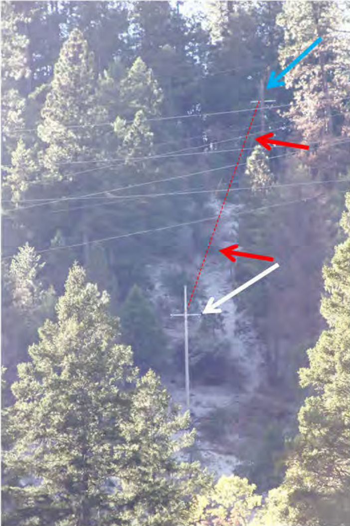
Figure 22: View of the line from Cresta Dam. The white arrow shows approximately where the tree fell adjacent to Pole 100403909. Pole 100403908 that supported the fuses is at the top of the hill (blue arrow). The cable PG&E installed between the two poles is the white line directly below and to the right of the dashed red line and is indicated by two red arrows.
