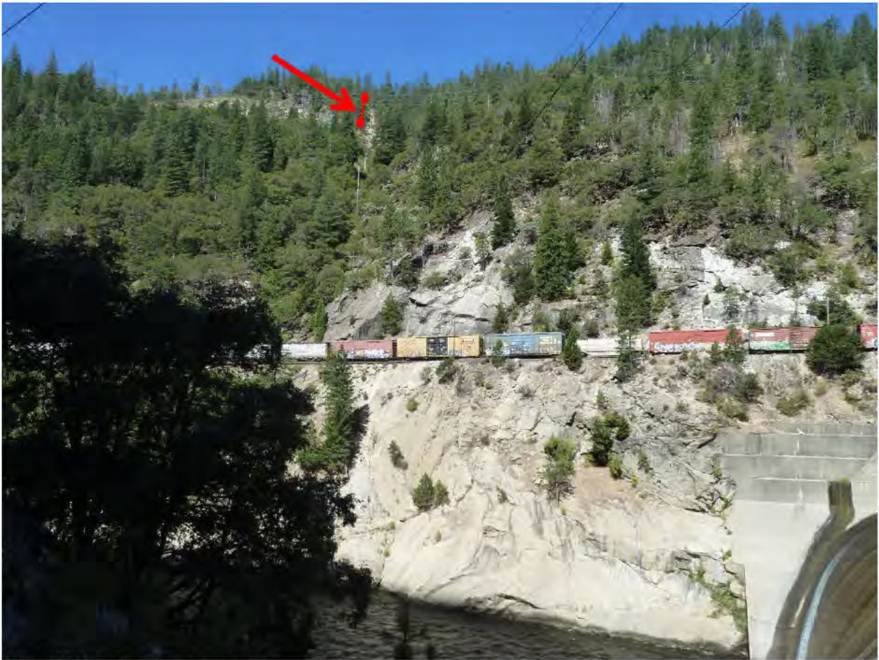
Figure 29: This photo was taken on November 13, 2014 (per the photo's metadata). The span of interest is highlighted with the red arrow. The red line shows the length of the span. The top oval connected to the red line is adjacent to Pole 100403908 which supports Fuse 17733. The bottom oval connected to the red line is adjacent to Pole 100403909, which is closer to where the tree rested after falling onto the line. The photo was taken as part of a pole replacement project at a pole lower down the hill.
