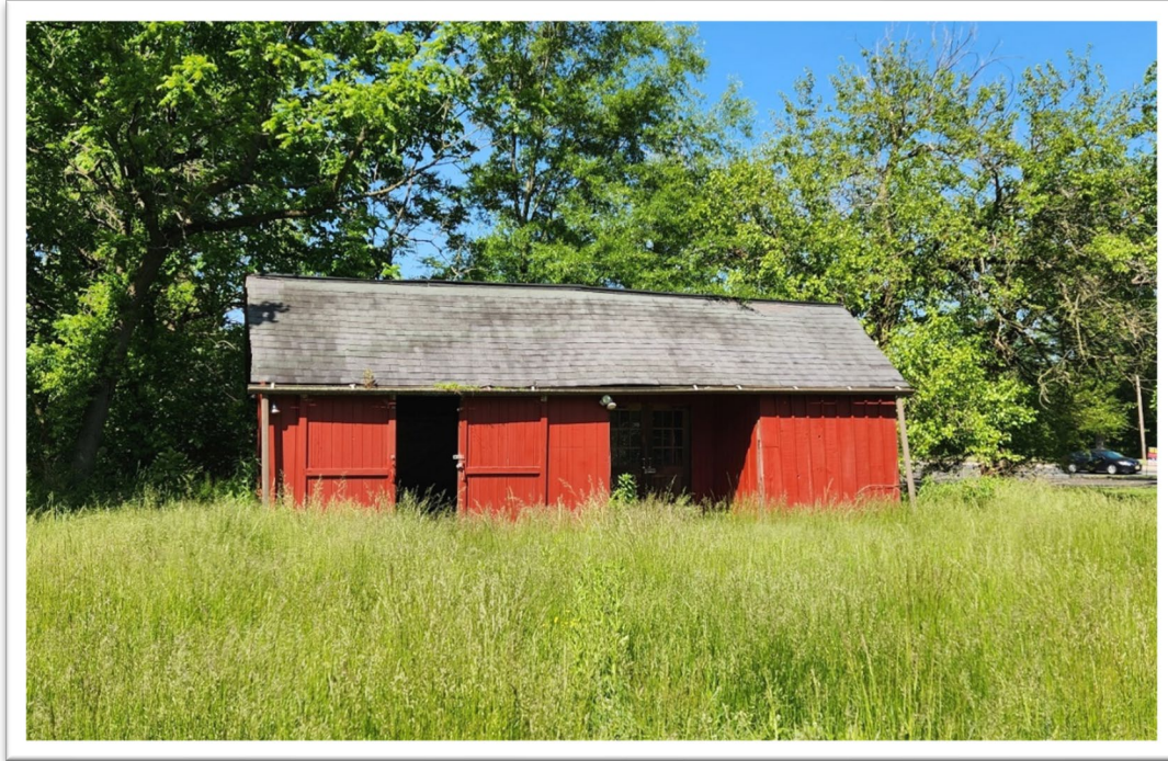
Figure 4 – Accessory Barn Structure
