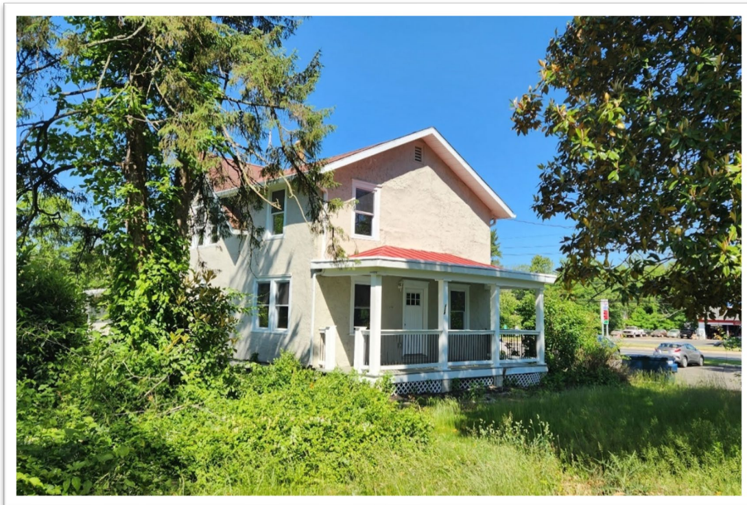
Figure 3– Vacant house with overgrown vegetation
