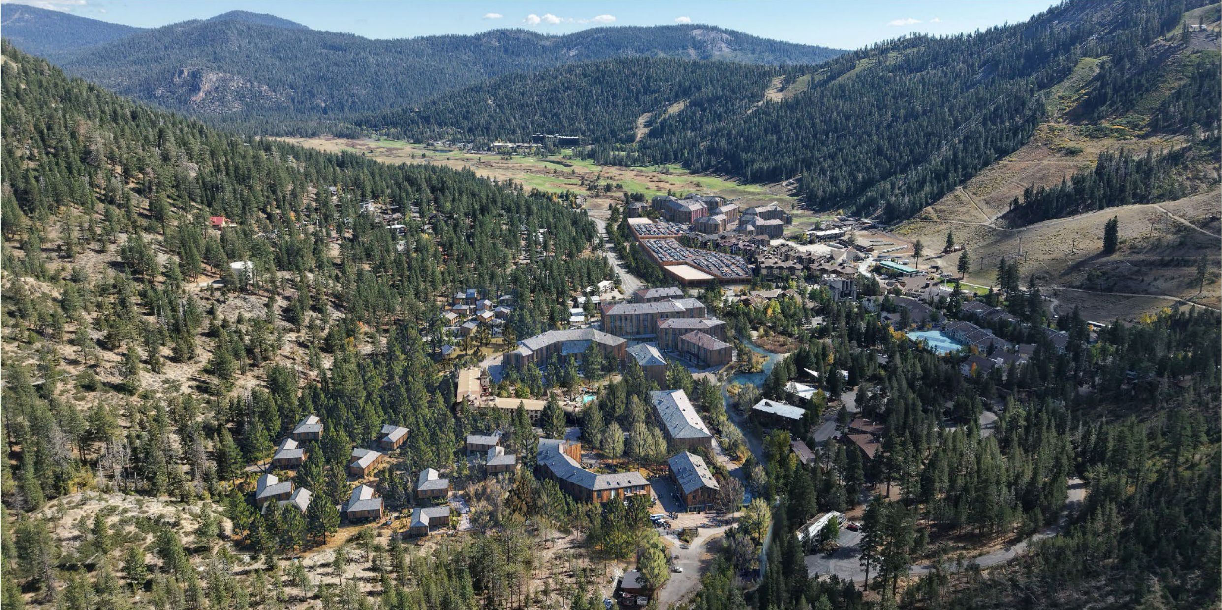
THE VILLAGE AT PALISADES TAHOE SPECIFIC PLAN Note: This illustration depicts a representative design that conforms to the Specific Plan's zoning and design standards. Actual building placement and design may differ. B-4
