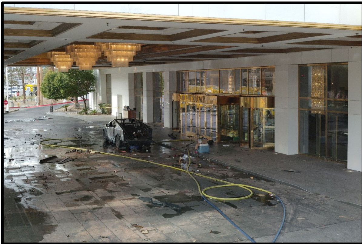
Figure 4. LVMPD Drone Photo of the Cybertruck in the Trump International Hotel Valet After the Fire Was Extinguished
