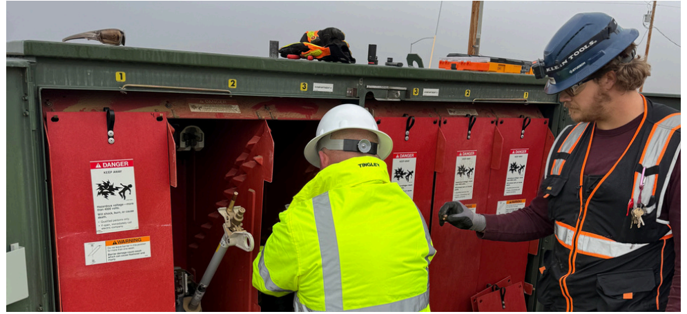
Left: a worker from Ardent dons protective electric work gloves in order to safely flip the main electrical switch, a task entailing 24,900 volts. Right: workers from Target Construction and Ardent are pictured safely making final electrical connections at the WFH Main Electrical Switch.
