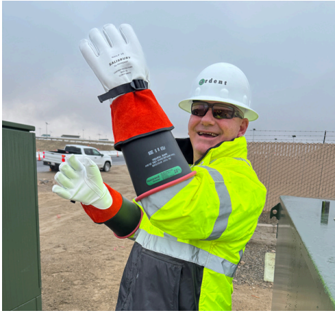
Left: a worker from Ardent dons protective electric work gloves in order to safely flip the main electrical switch, a task entailing 24,900 volts. Right: workers from Target Construction and Ardent are pictured safely making final electrical connections at the WFH Main Electrical Switch.
