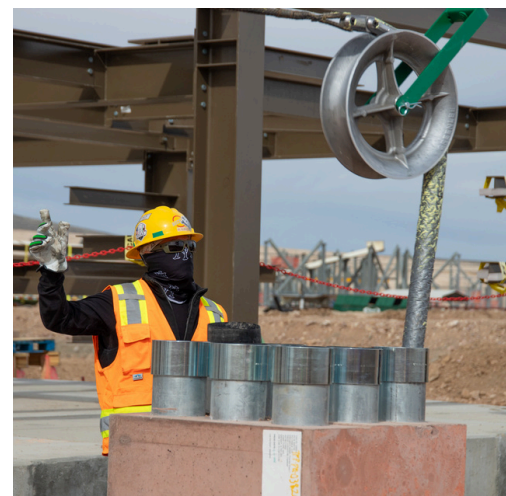
The first aboveground pipe installed: a 288-pound carbon steel section was craned into the Filter Building in late January 2026.
