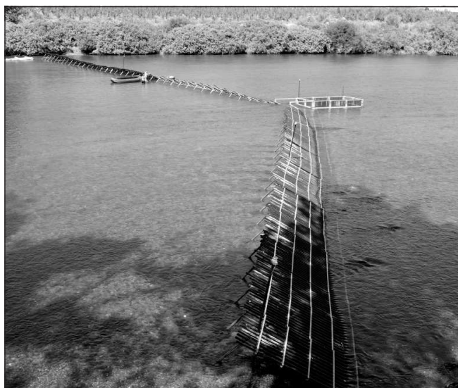
MICHELLE CAMPOBASSO/CTFW The weir just south of Malott Bridge during construction.
