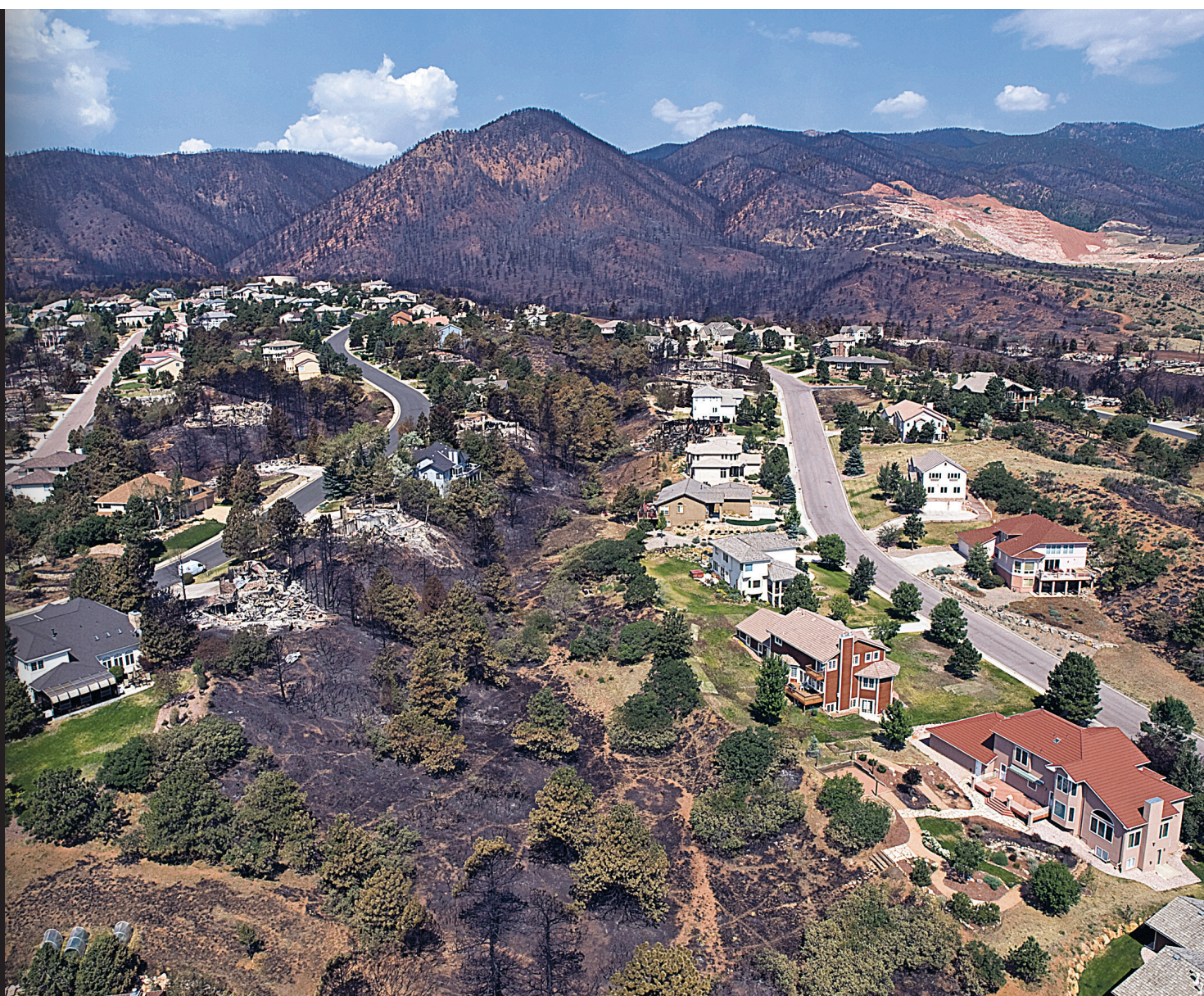
The Waldo Canyon Fire burned 18,000 acres and more than 350 homes in Colorado last summer. A new assessment shows many more houses and properties would have been destroyed if the communities had not worked to reduce wildfire risks. PHOTOS COURTESY KARI GREER/U.S. FOREST SERVICE
