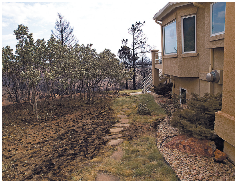
A properly built structure and defensible space helped one house survive the Waldo Canyon Fire in Colorado Springs, Colo.
