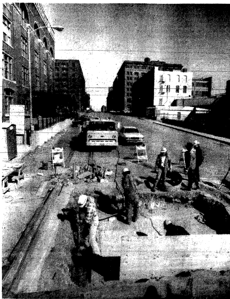
Omaha Public Power District workers at Ninth and Jackson Streets ... Increased electric power is part of the improvements to the redevelopment area.
