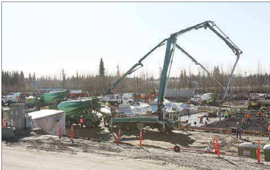
The concrete slab is poured at the site of the new UAF Heat and Power Plant off of Alumni Drive on Thursday morning. Three concrete companies hauled in 1,764 cubic yards of material in 25 truckloads, with 45 workers on the ground leveling the five-foot-thick slab. The new heat and power plant has an estimated cost of $245 million and a completion date of 2018. ERIC ENGMAN/NEWS-MINER PHOTOS
