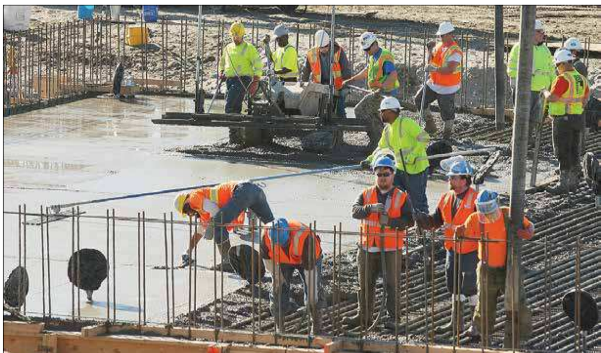
The concrete slab is poured at the site of the new UAF Heat and Power Plant off of Alumni Drive on Thursday morning. Three concrete companies hauled in 1,764 cubic yards of material in 25 truckloads, with 45 workers on the ground leveling the five-foot-thick slab. The new heat and power plant has an estimated cost of $245 million and a completion date of 2018. ERIC ENGMAN/NEWS-MINER PHOTOS
