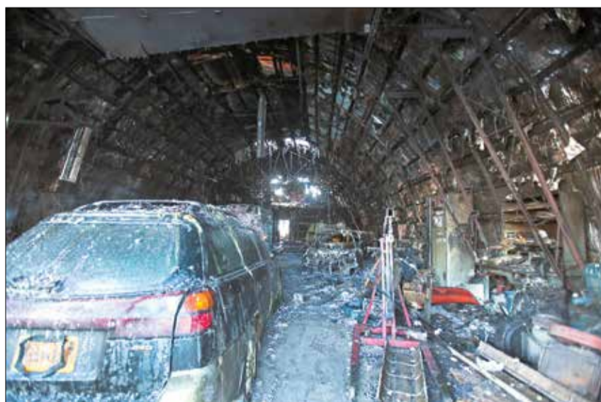
The burned out remains of Jim's Auto Parts & Glass seen on Friday. A gasoline leak from a vehicle under repair caused the fire that destroyed the auto and glass shop and attached home Thursday, according to a Fairbanks fire official. ERIN CORNELIUSSEN/NEWS-MINER
