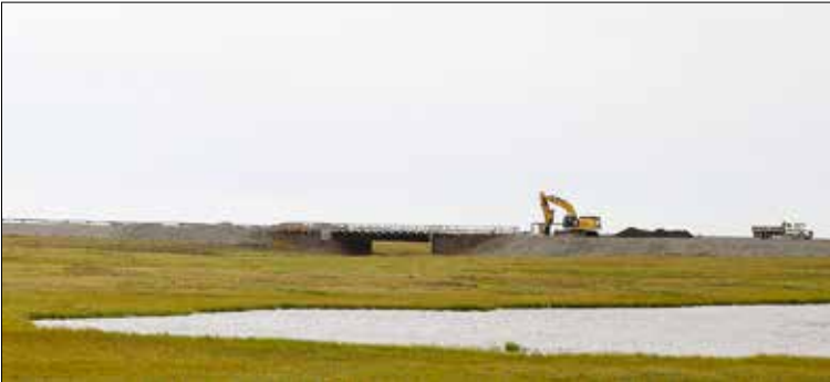
A backhoe works on gravel slopes surrounding a bridge on Thursday. ERIN CORNELIUSSEN/NEWS-MINER
