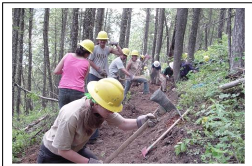
Constructing new trail
