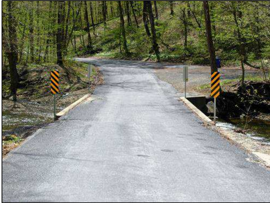
Photograph No. 1. Approach from East - Looking West
