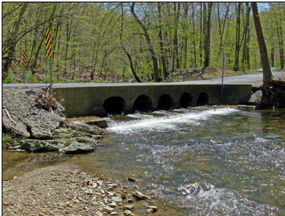
Photograph No. 4. Downstream Elevation
