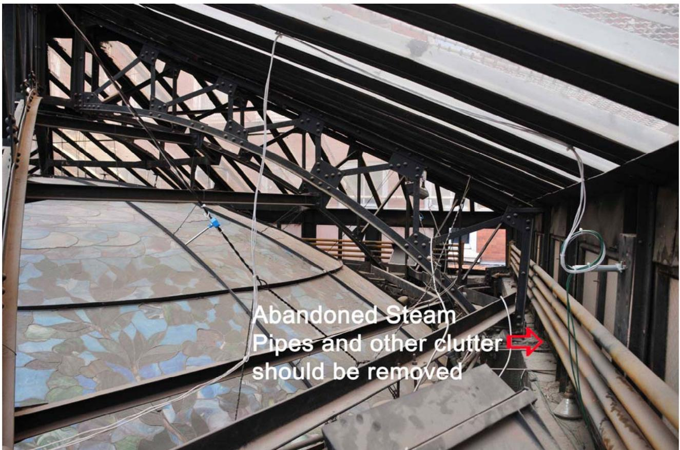
FIG 6. Interstitial space between the domes; abandoned steam radiation pipes on the right.
